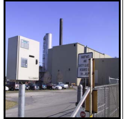
Scale lane automation for facilities using the WasteWORKS software package.
