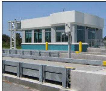
Brevard County's new, state of the art transfer station facility, the Melbourne transfer station opened for operation just weeks before facing Frances.
