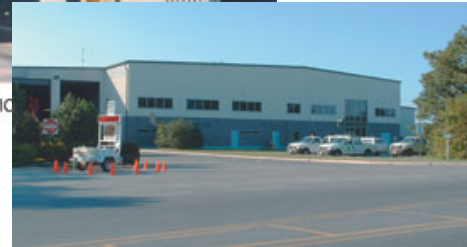
PHOTO: ATLANTIC COUNTY UTILITIES AUTHORITY
